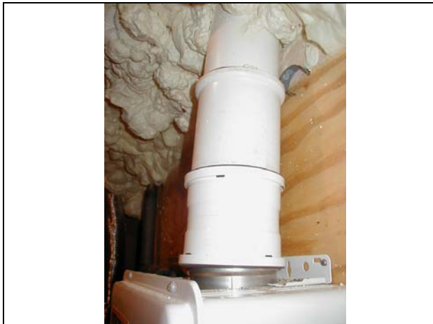
Rinnai sealed combustion through foam
