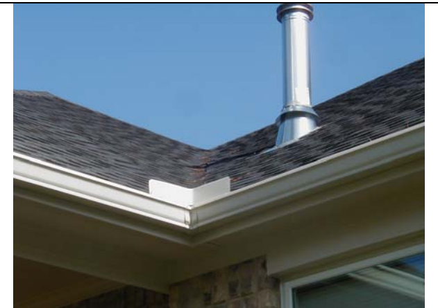
Rinnai flue on roof
