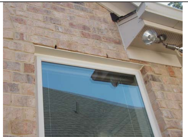
Weep hole over window
