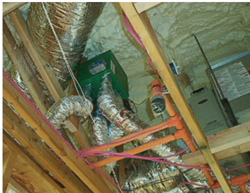
Supply air distribution ventilation system located in attic space distributes outdoor air to four rooms in the home at volumes that do not adversely affect comfort.
