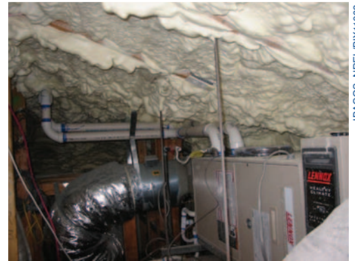
Air-handling units in attic space are protected from outdoor conditions and can operate more efficiently.
