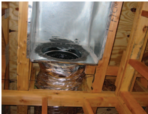
Extensive efforts were made to seal the air distribution system against air leakage.
