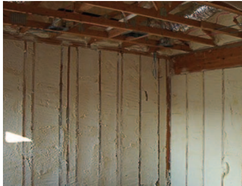
Spray foam insulation used in exterior walls.
