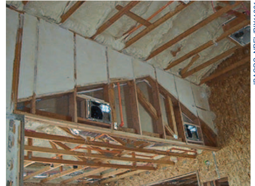
Spray foam insulation used at the underside of roof sheathing at two locations.
